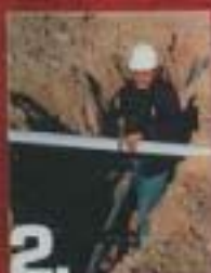
STEP 2: Cut Split Duct Conduit to Fit
